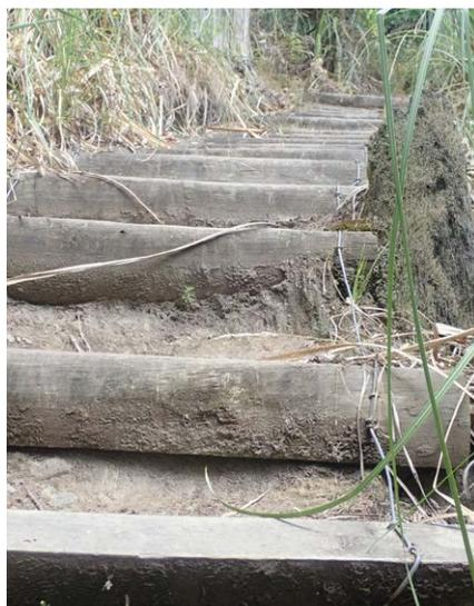
Warren Geraghty steps on the Lipsey track on Mt Te Aroha. These are constructed off site from half rounds and #8 wire and then rolled up for carrying to slopes to where they are needed. Over time they embed themselves into the slope and have a long life as steps. Warren Geraghty was a forester who later in life worked for DOC in this area for many years. Photo: Julia Stace.
